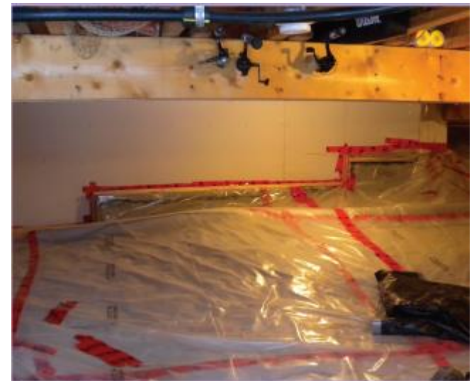
Membrane installation
