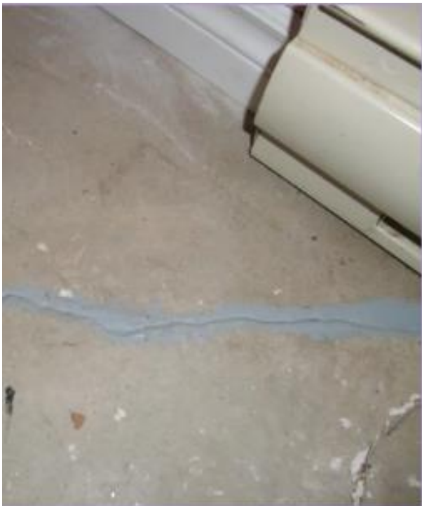
Floor crack seal
